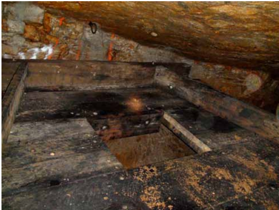
Construction of Ore Chute at base of the Dickenson's Stope (4L).
