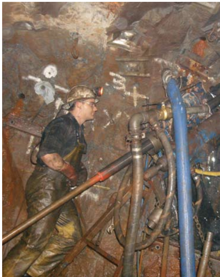
Drilling at Morning Star's Victorian tenements
